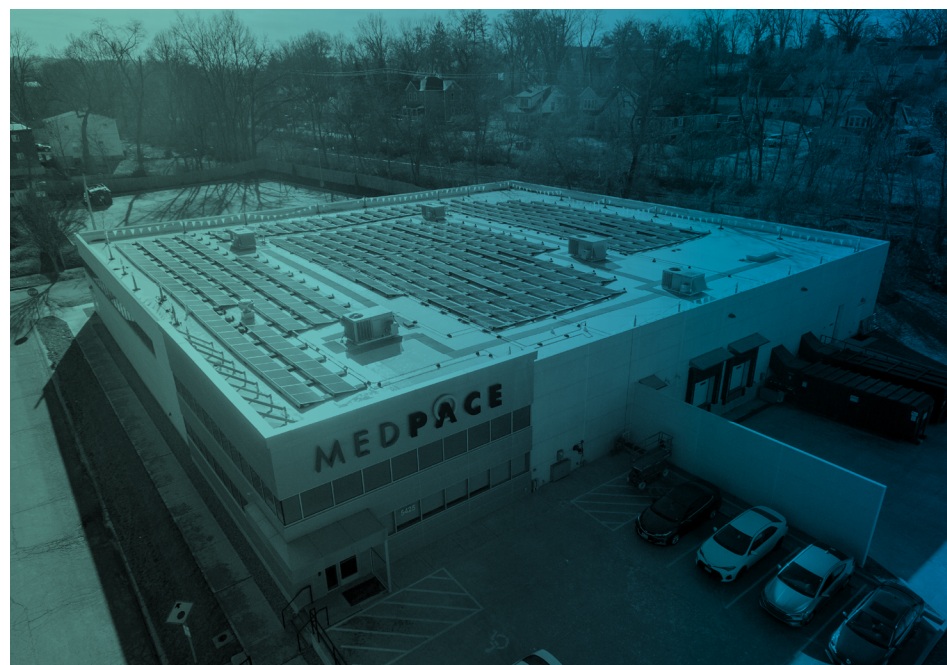
One of four buildings with solar panels on Medpace's campus
